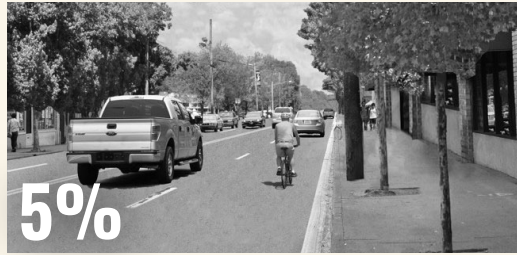
No bicycle facility on a four-lane roadway.
