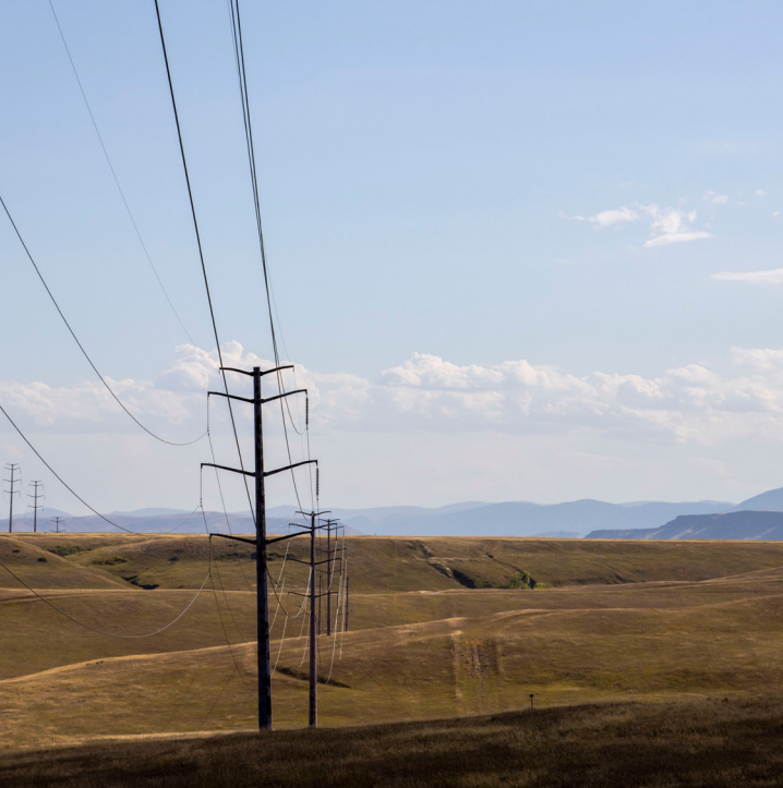
Electricity transmission lines.
