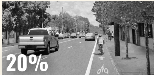
Bicycle lane on a four-lane roadway.
